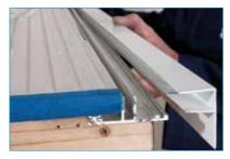
Finish the edge of the roof with an F-profile which can be secured to the rafter or barge board with screws.
