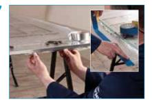
Fix the sealing tape at the top end of each piece of Corotherm and the perforated breather tape at the bottom making sure tapes are not creased or torn.
