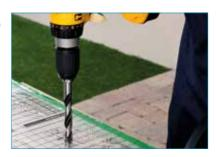
Remove the sheet to the bench to drill where you have marked. Remember all Corotherm sheets must have an expansion allowance of 3mm around all fixings.
