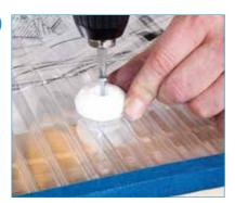
With the sheet now in the correct position, secure into place using the Corotherm fixing button in the pre-drilled hole. Flashing tape forms a completely watertight seal at the top of the sheet.
