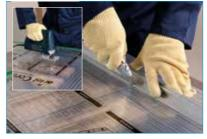
When cutting parallel to the flutes a sharp knife can be used but when cutting across the flutes a fine toothed saw is required. For cutting curves use a fine-toothed jigsaw.
