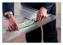
Any swarf from cutting or drilling should be removed by vacuuming. Next peel back the protective film from all edges of the Corotherm sheet on both sides
