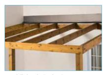
Pre-drill the glazing bar in preparation for fixing to the rafters - at approximately 400mm centers staggered on alternate sides.
