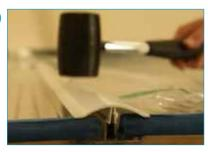
Starting at the downslope end, line up the ends of the cap and base and tap home with a rubber mallet until the edge seals have flattened against the sheet.
