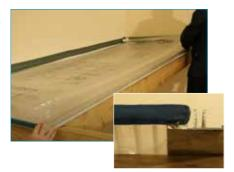
With the silver sealing tape at the top of the slope and the breather tape at the bottom, push the sheet into position between the glazing bars. Ensure that the printed film is facing upwards. At least one vertical rib of each Corotherm sheet should engage with the glazing bar at each side, again leaving a 3mm expansion gap.
