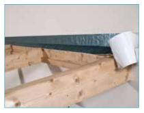
Begin the project by installing the flashing tape to provide a watertight seal between the wall and roof.
