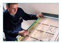
Set the correctly sized sheet into position allowing a sufficient expansion gap at the top end of the sheet and mark a hole centrally at the lower end of the sheet for a fixing button. This fixing will prevent the sheet from moving once installed.
