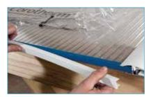
To protect the breather tape, fit end caps or U-profiles to the end of the sheet.
